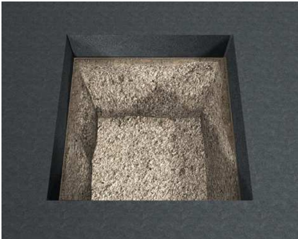
Figure 8. Remote asphalt and aggregate to create a hole.
