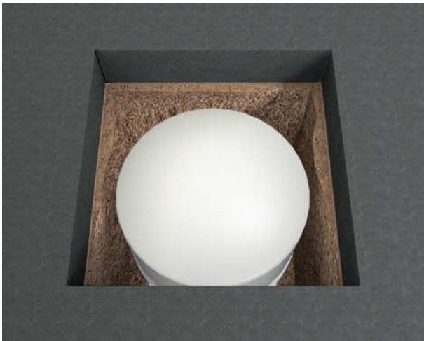
Figure 9. Place the PVC enclosure into the hole.
